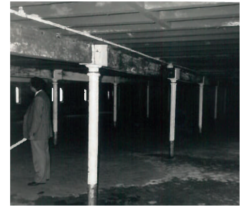
Figure 12 A photograph taken in 1991, showing the interior of the maltings, with cast iron columns, a floor surface of setts and timber structure of the first floor (Essex County Council)
