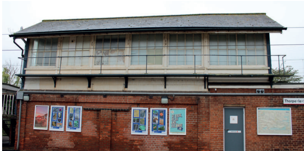
Figure 20 The signal box on Thorpe-le-Soken's island platform
