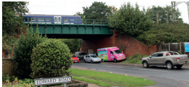
Figure 21 Thorpe-le-Soken railway bridge
