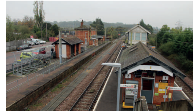
Figure 37 Viewpoint 2 looking east from the station footbridge
