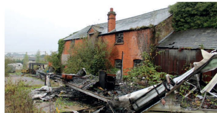
Figure 49 The stable and coach house building
