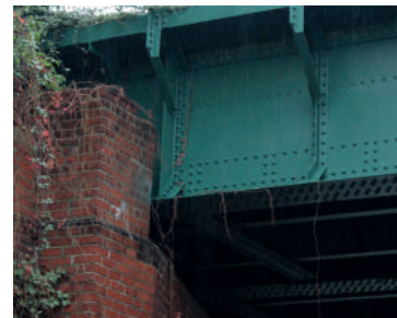
Figure 22 A detail of the railway bridge
