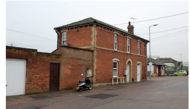
Figure 18 A photograph of the station master's building today after refurbishment and reuse as two residential properties
