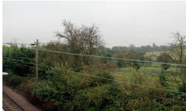
Figure 36 Viewpoint 2 looking south from the station footbridge
