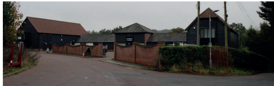
Figure 26 The commercial buildings built on part of the former market site
