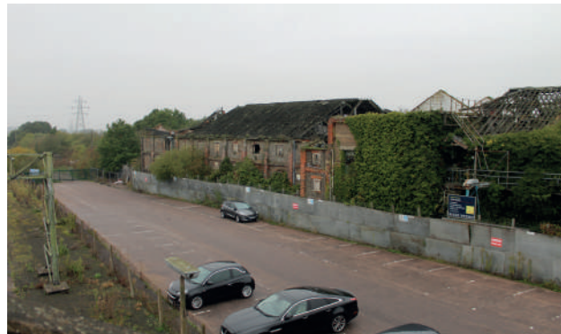
Figure 39 Viewpoint 2 looking north-west
