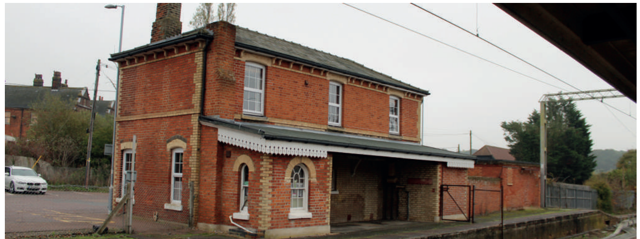
Figure 19 The Station Master's House looking northeast from the active station platform
