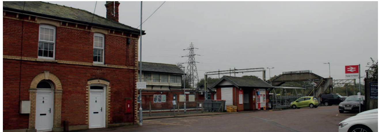
Figure 25 The station Masters House with the signal box of Thorpe-le-Soken station behind
